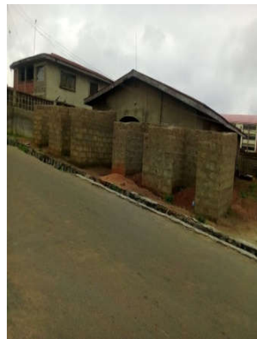
Plate 2: on-going construction of shops on Olubuse Street Source: Fieldwork, 2019
