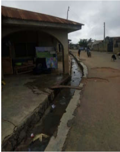
Plate 3: Residential real estate project on Olubuse Street Source: Fieldwork, 2019
