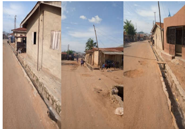
Plate 6: Residential real estate project on Olubuse Street Source: Fieldwork, 2019
