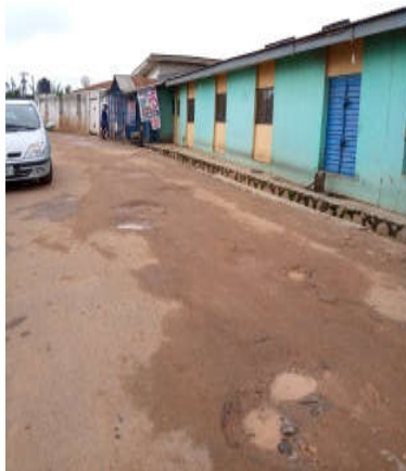
Plate 5: Residential real estate project on Olubuse Street Source: Fieldwork, 2019
