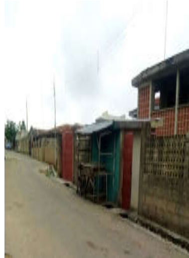
Plate 4: Residential real estate project on Olubuse Street Source: Fieldwork, 2019
